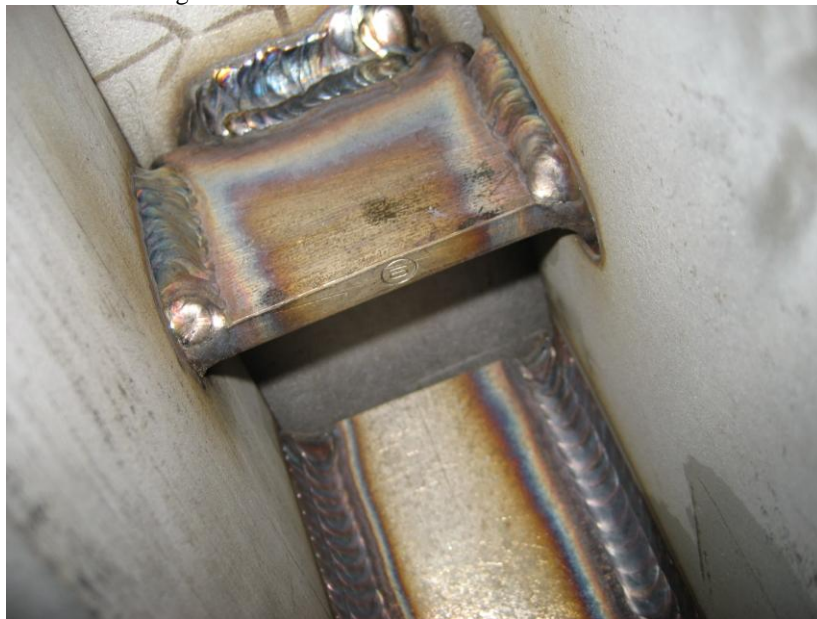
Figure 5.4-2 Photo of the One of the Tabs that Connect Rib Pairs
