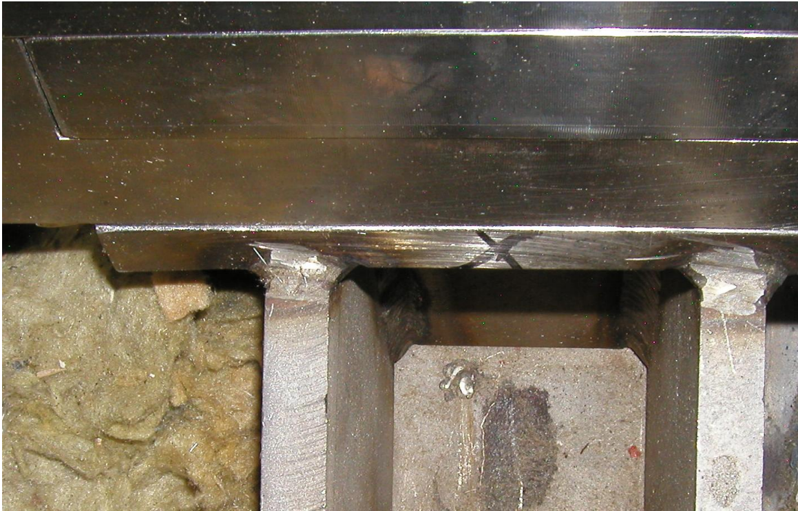
Figure 9.3.4 Area Recommended for Inspection
